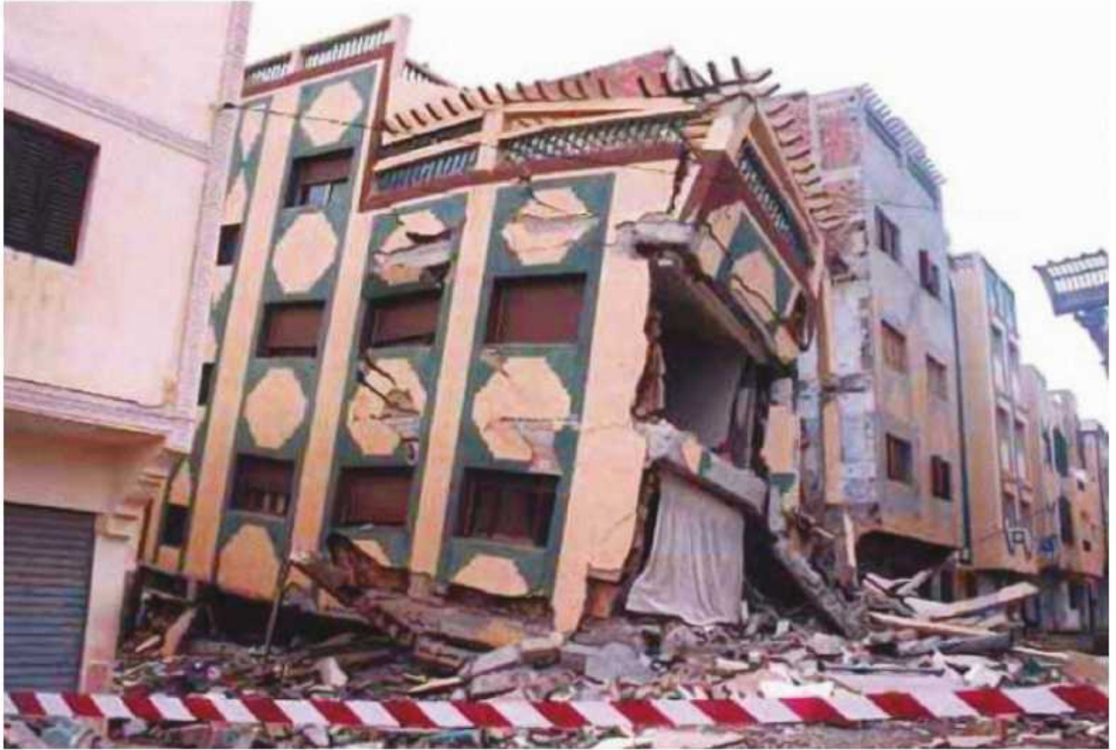
Figure 2.7: Damage caused by the M6.4 earthquake that struck Al Hoceima, Morocco on 24 February 2004. 38
