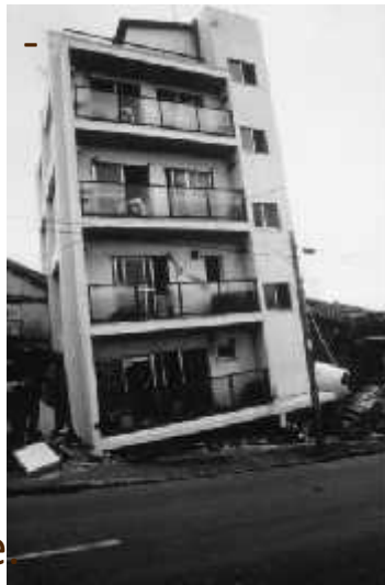
Class #8 - reinforced concrete shear wall, without moment resisting frame, medium rise
