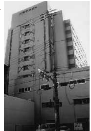
Class #9 - reinforced concrete shear, wall without moment resisting frame, high rise
