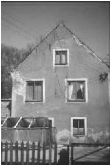
Class #3 - unreinforced masonry, with load bearing wall, low rise.
