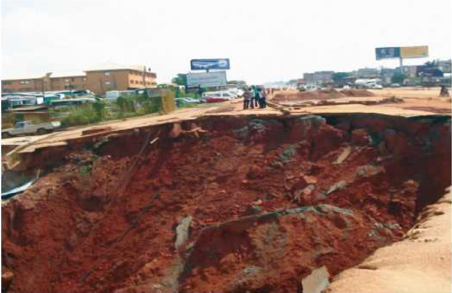
Figure 5.3: Mass movement affecting express highway in Onecha City, Nigeria, which is associated with gully erosion development.
