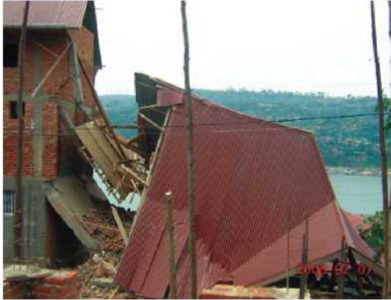
Figure 2.9: Damage in Bukavu, DRC, caused by the M_w 5.9 earthquake that struck the Lake Kivu region on 3 February 2008. 45
