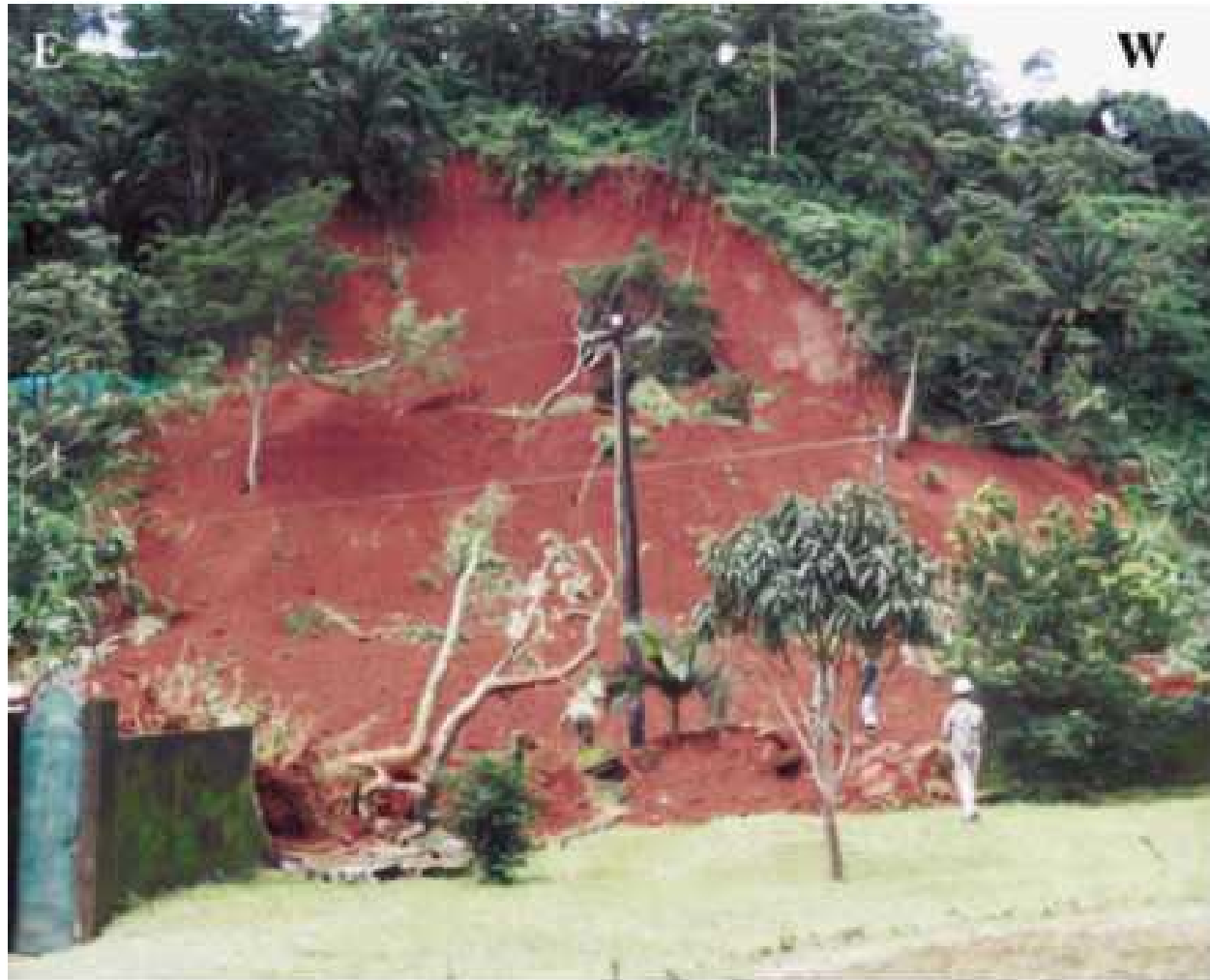
Figure 5.4: View of a rotational landslide at Kie Village developed on weathered pyroclastic cone characterised by reddish to reddish-brown soils. The green structure at the centre-left edge of the picture is a 300 m 3 water tank, which is partially buried by slide debris 44 .
