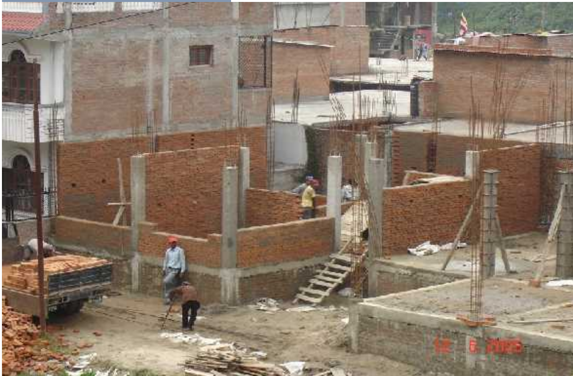
Reinforced concrete frame building with brick infill walls under construction, Kathmandu, Nepal (© J. Bothara)
